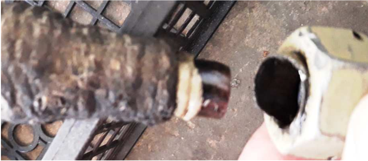
Fitting on the oil pump (to oil filter) was broken. The fitting was loose and there was a plastic cover foil on the fitting over the throat.
