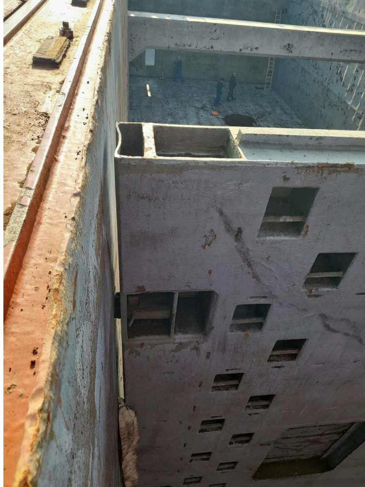
Image 3. Moveable bulkhead installed in cargo hold with transverse fastening pins
